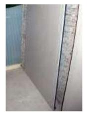
Panels of Spaceloft 9251 laminated to building facing board were easily attached to apartment walls and around windows and other fixtures (above).
