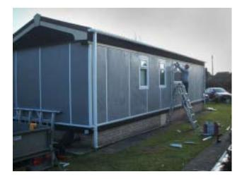
ParaClad<sup>™</sup> panels with Spaceloft 9251 were easily installed on the exterior of the mobile home.
