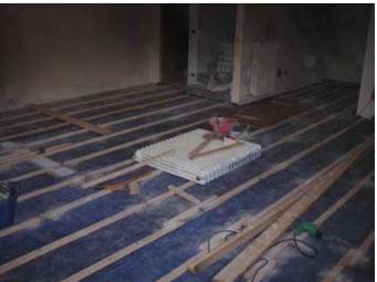
It took just 30 minutes to install Spaceloft 9251 throughout this entire room. Polystyrene foam takes a full day to install. The aerogel insulation dramatically improved the thermal comfort of the floor.
